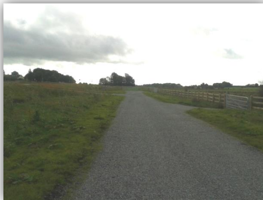
Figure 1-3: Example of a Typical Access Track.
